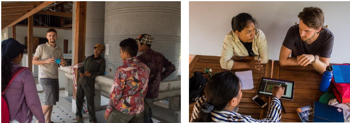
Figure 5: Left: Fridolin Tschudi explains how to connect PVC pipes for the newly built hatchery. Right: Silvan Oberhänsli, Sreymom Y and Theory Soeun during a scheduled team meeting.
